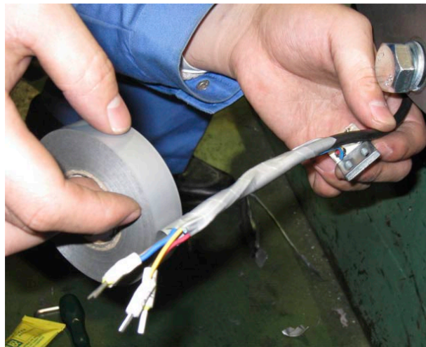
Figure 31 Wrap with electrical tape
